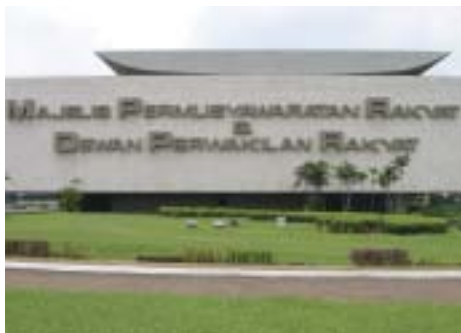
Strengthening the House
